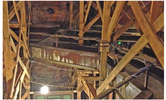
Scaffolding supports the balcony and roof.
