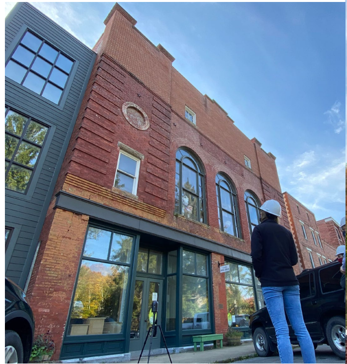
The Mills Group surveying the Opera House in fall of 2020
