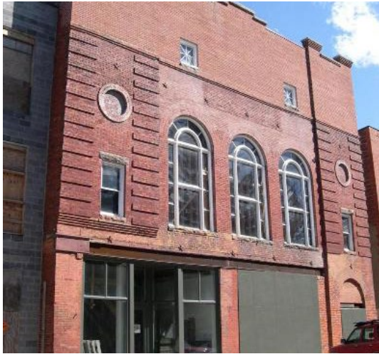
Ongoing stabilization work in 2008
