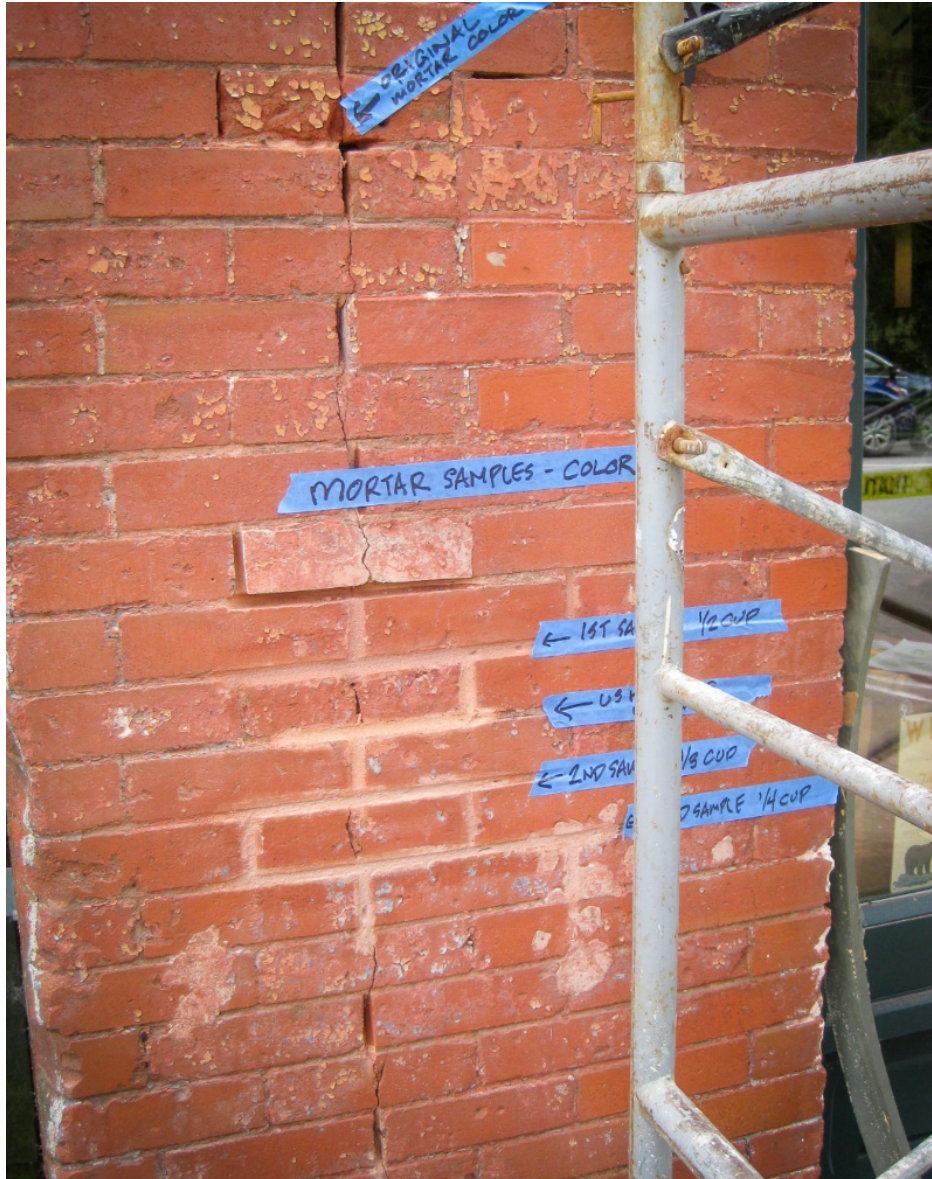
Samples to match the original mortar from 1902.
