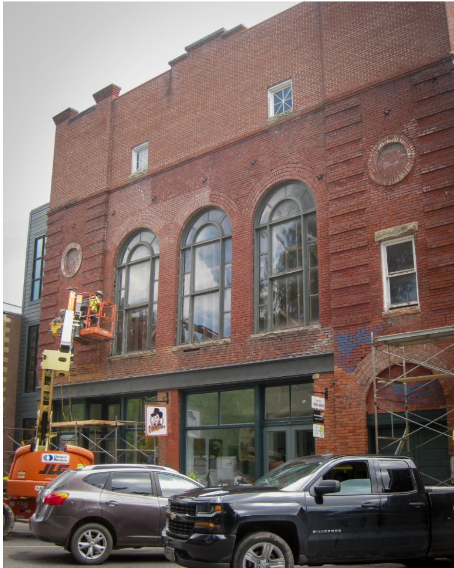
The Opera House during brick restoration in 2021.
